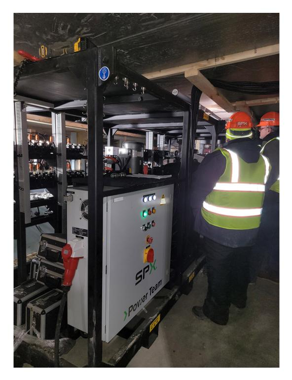
After demolition, from the ground to 16th floors, they retained certain areas of the floor plates to meet the remaining retained slab requirement. The team also added a subcellar to the basement, removed the theater's old foundation and created new foundations, and put the hydraulics in place and a 5-ft ring beam around the perimeter of the theater -- "all with 16 stories above our heads," Israel says.
