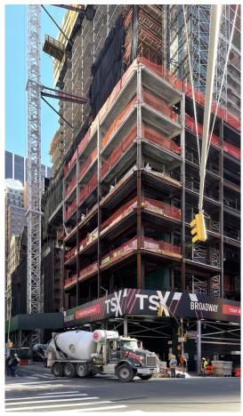
The reinforced concrete core is positioned along the southern section of the building's footprint, as seen when looking north on Seventh Avenue from West 42nd Street. The string of punched-out window openings among the flat concrete surface is starting to stack up with each newly completed level.
