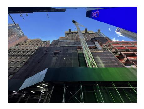
There are several new hotel floors constructed atop the intricate system of diagonal steel columns and trusses connecting to the multi-story podium. The steel work continues to be fireproofed and will eventually be covered in a massive wraparound LED screen similar to the one that was designed for the Times Square EDITION across West 47th Street.
