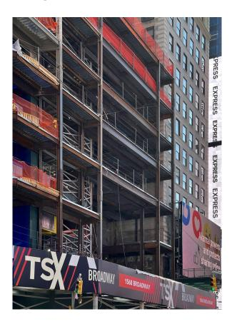
The safety cocoon system and concrete form work are rapidly helping to create the tower. We can also start to see more of the rounded northern corner.
