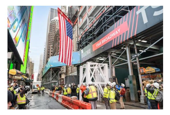
At the beginning of 2022, construction teams began a delicate, multi-phase integration of the existing Palace Theatre. Led by PBDW Architects, this involves raising the venue with massive hydraulic lifts installed beneath the foundation. The building's hotel volume will be built around the theater and a new retail corridor installed below.
