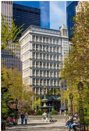
195 BROADWAY. PHOTO: L&L HOLDING COMPANY
