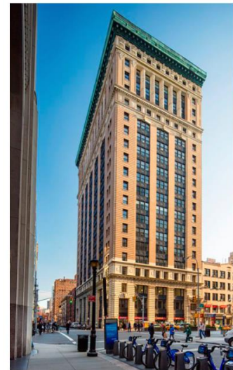
315 Park Avenue South
