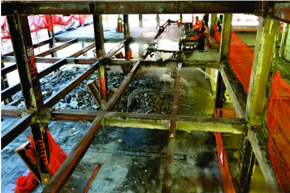
Structural work at 390 Madison Avenue, photo via L&L Holding
