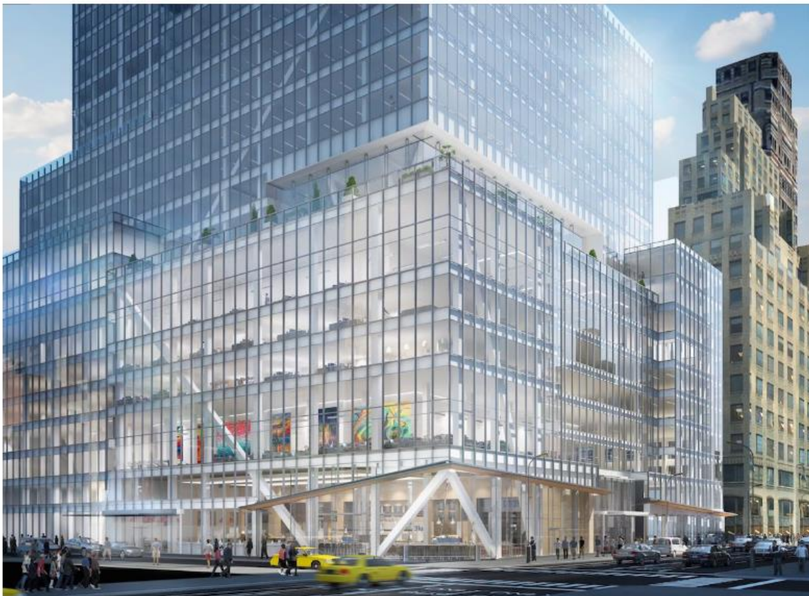
The double-height entrance and lower floors of 390 Madison, via L&L Holding
