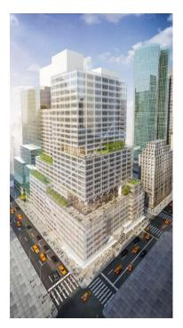
The heart of the renovation project centers on the re-massing of the property, with millions of pounds of steel and concrete removed from the base of the building and replaced with eight new floors at the top. Last year, the building completed its structural transformation, increasing the old 24-story structure by 108 ft. to its new height of 32 stories and 373 ft.
