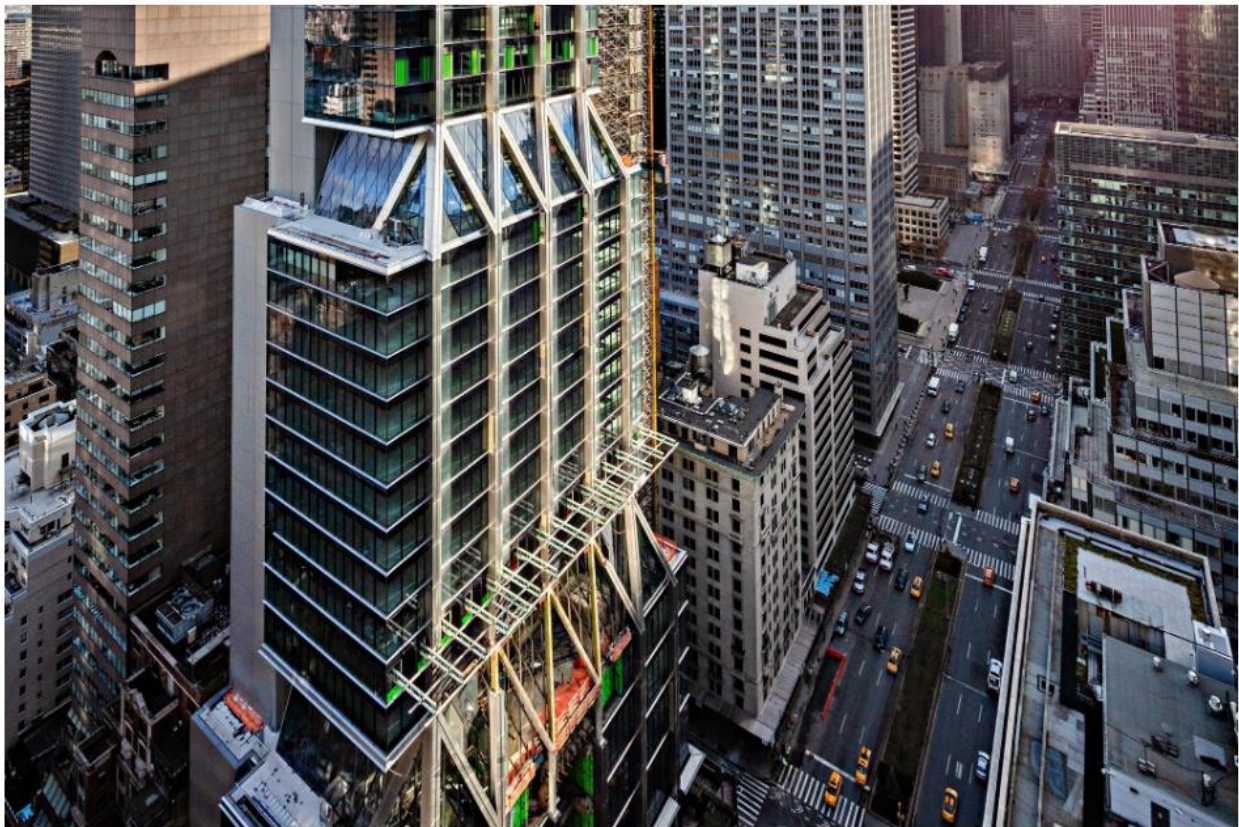
L&L Holding Co. is nearing completion of its 47-story New York office tower, 425 Park Avenue. (Alan Schindler/L&L)
