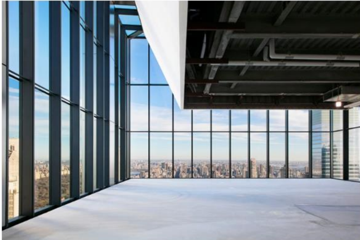
Interior Construction at 425 Park Avenue – Photo by Connie Zhou
