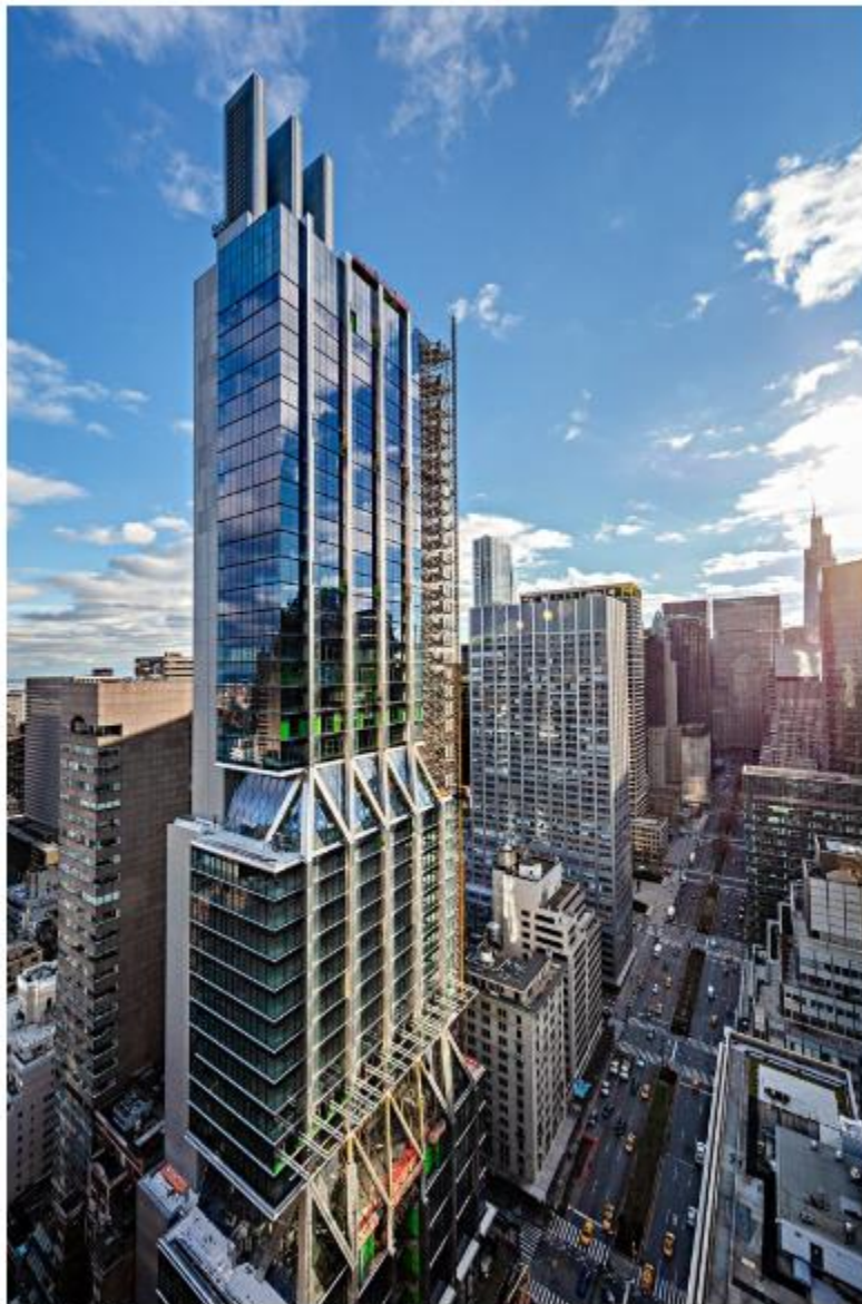
Exterior View of Construction at 425 Park Avenue - Photo by Alan Schindler
