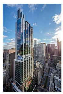
The building's crowning jewel – a set of three distinctive ornamental fins that will be illuminated via LED technology – has been fully constructed and clad in steel and glass atop the 897-foot tall tower. At street level, 425 Park's grand 45-foot tall lobby, featuring stone flooring, interior glass walls, modern lighting and state-of-the-art elevator systems is also nearing completion.
