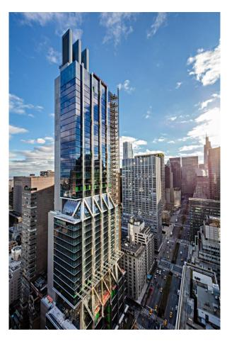
According to a press release, the glass-and-steel facade is now fully enclosed, the ornamental fins have been fully constructed, and the exterior tower crane has been dismantled and removed. In addition, the building received a temporary certificate of occupancy, which means that as soon as the project is complete, tenants can begin moving in.
