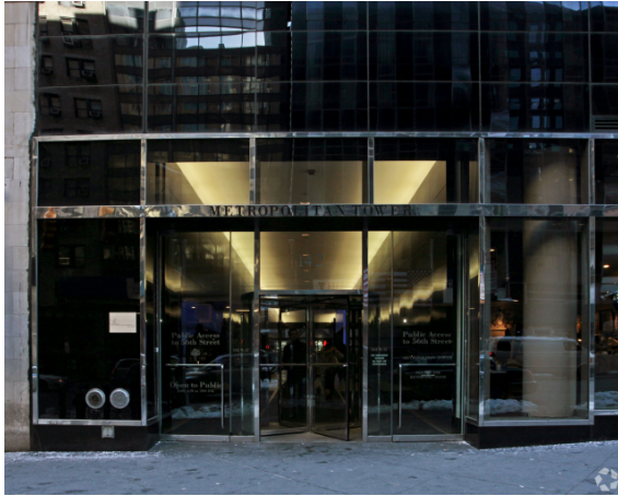
METROPOLITAN TOWER AT 142 WEST 57TH STREET (PHOTO: COSTAR).
