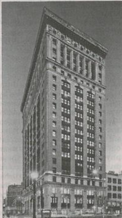
315 Park Avenue South
