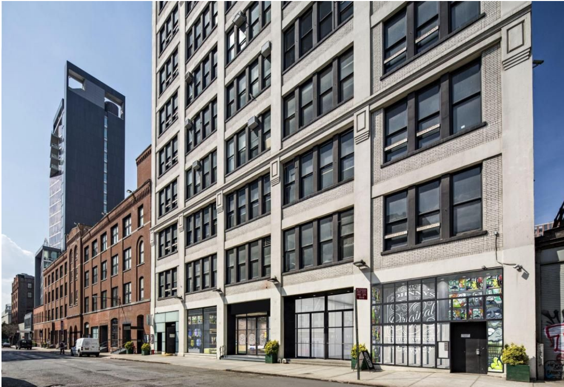
Courtesy: L&L Holding Co. 85K SF office building The Ironworks at 511 West 25th St.
