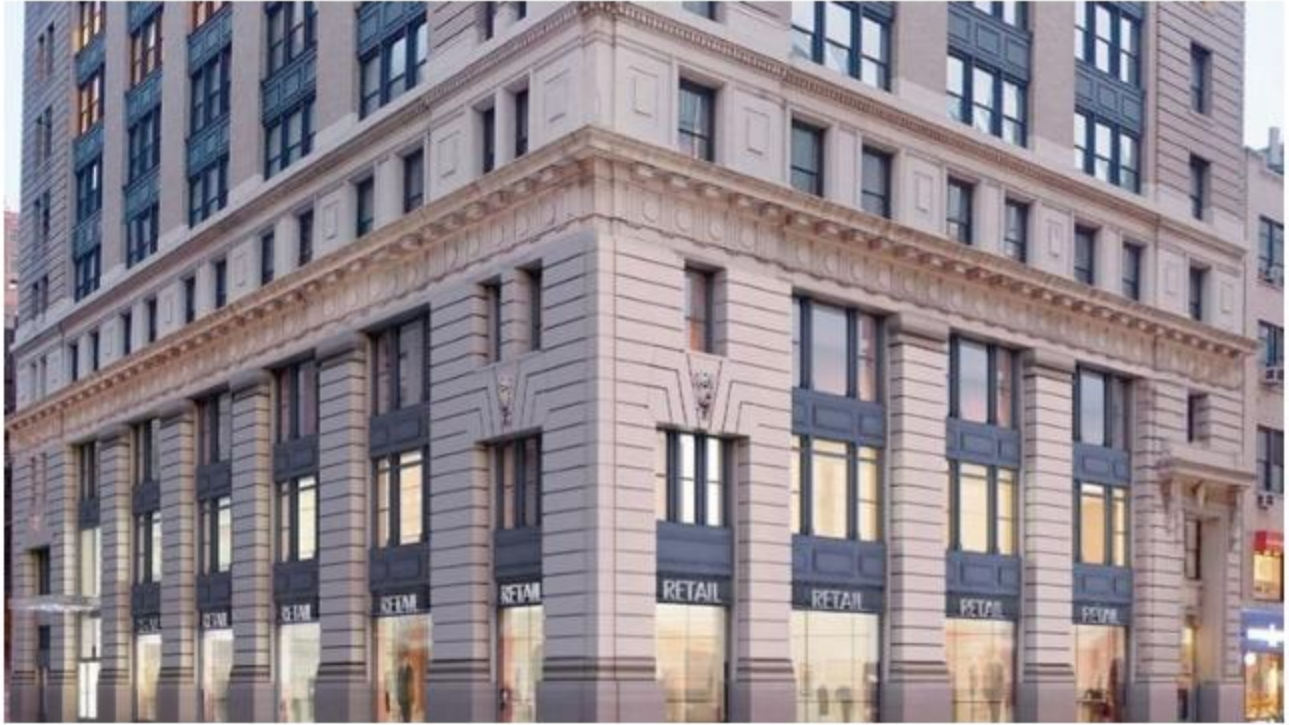
Columbia Property Trust is renovating the 20-story building at 315 Park Ave. South.
