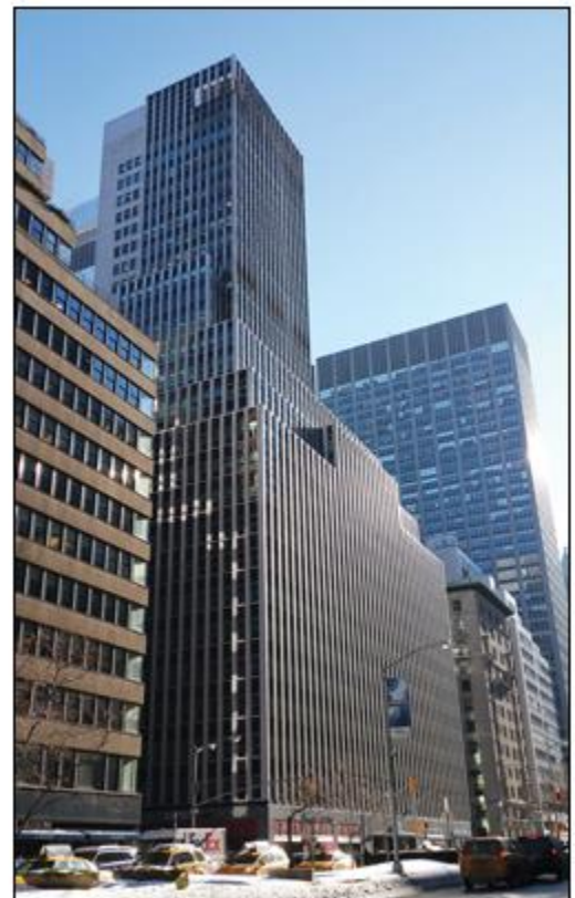
425 Park Avenue before construction started
