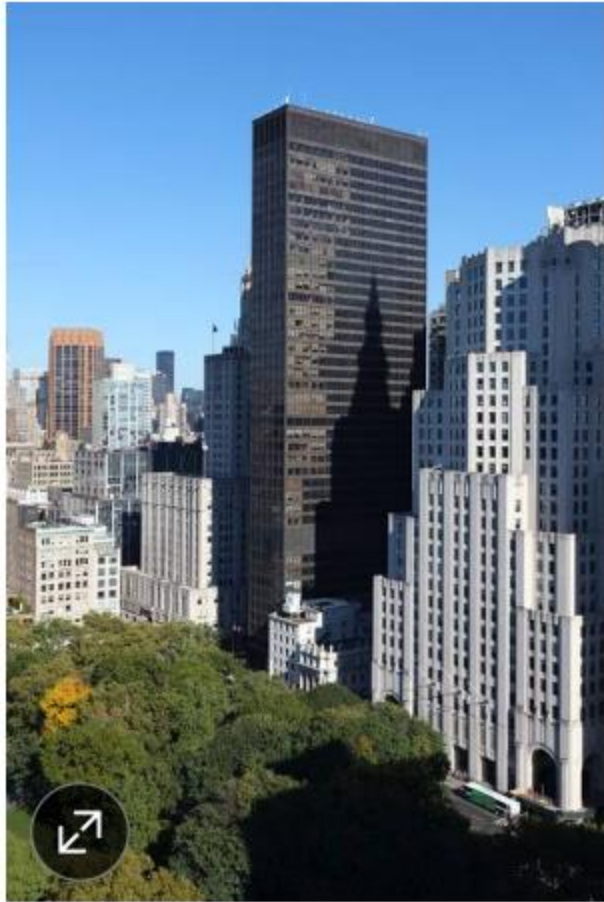
Rudin Management is investing about $15 million in renovations to 41 Madison Ave.
