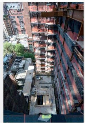
WORKERS DEMOLISHED THE BACK PORTION OF THE BUILDING AFTER REMOVING THE 33RD TO THE 17TH FLOORS, PHOTO: ALAN SCHINDLER
