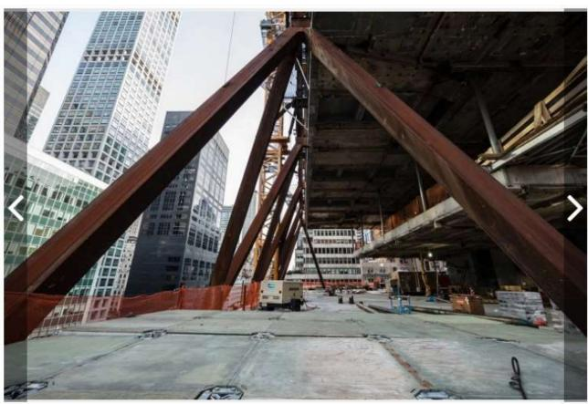
THE NEW STEEL COLUMNS WERE ADDED TO THE BUILDING AS THE OLD WAS BEING COMPLETED. PHOTO: ALAN SCHINDLER
